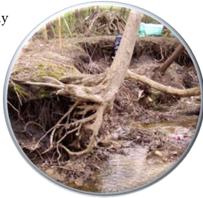
Severe streambank erosion (Source: Living Waters Consultants)
