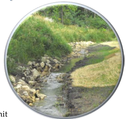
Streambank stabilization on Carpenter Creek
