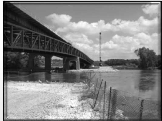
View of New pedestrian bridge for Stearns Road multi-use trail
