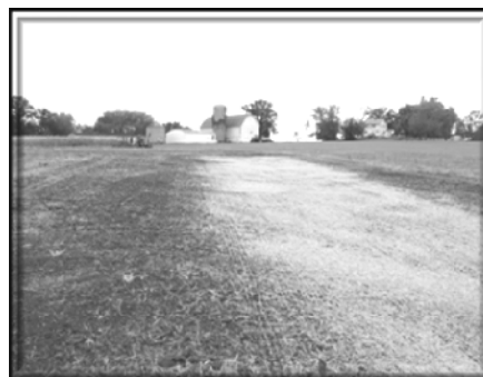
After: Grassed Waterway
