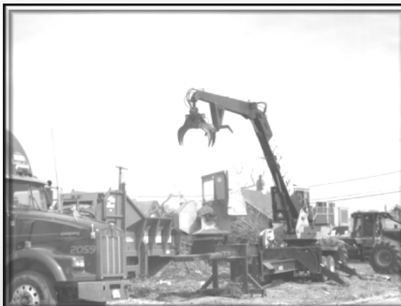
2010: Southwest Acquisition Area Demolition
